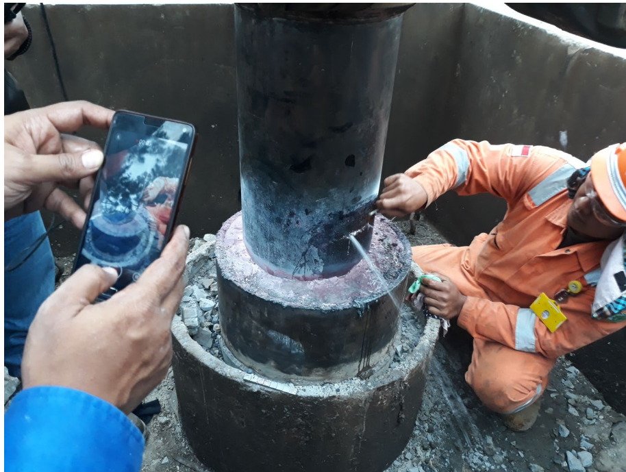
Figure 2. Crack in L-80 Casing / Weld Failure: Courtesy of PT TNG Energy Services Indonesia
